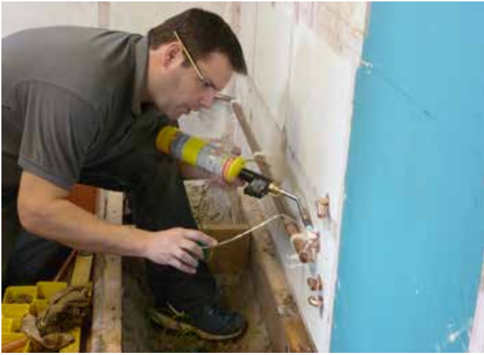
Russ- fitting the pipework.
