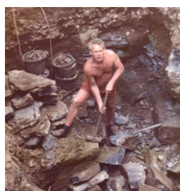
1978 DIGGING THE CESSPIT ? [?]
