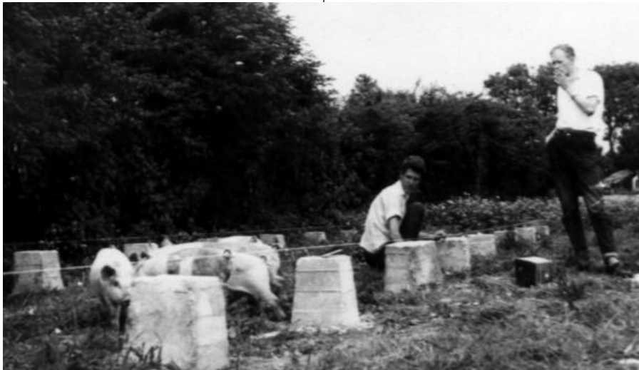
1964 COTTAGE FOUNDATIONS (AND PIGLETS!) [JOAN GODDARD]
