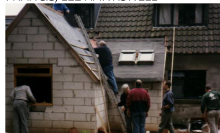
1997 ROOFING THE LIBRARY EXTEN- SION
