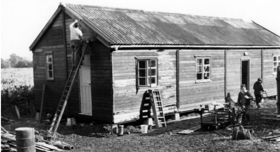
1964 THE ALMOST FINISHED WOODEN COTTAGE [TONY KNIBBS]
